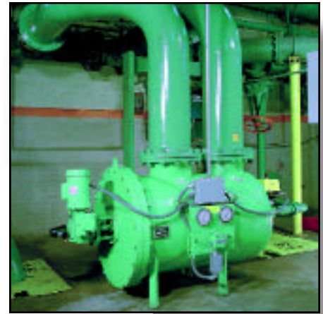
HWS Series Poro-Edge Strainer on river water supply to major tire manufacturing plant.
