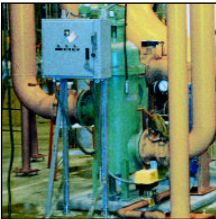
VWS Series strainer at automotive plant on broaching solution service.
